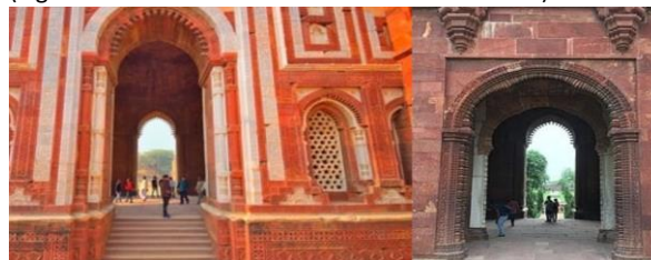
(Figure10A: Southern entrance and northern entrance)
