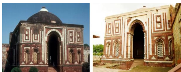
(Figure10B: Western entrance and eastern entrance)
