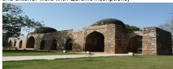
(Figure13: northwest rooms of Alai madrasa)
