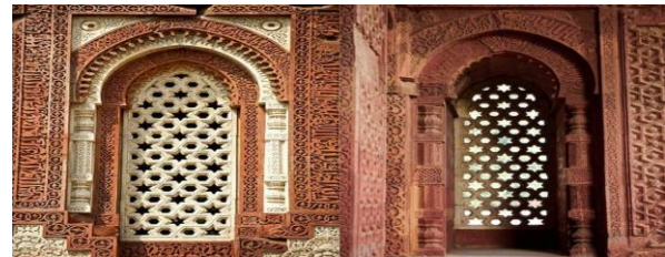
(Figure11: Latticework window on the both sides interior and exterior walls with Quranic inscriptions)
