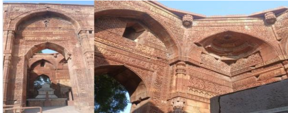
(Figure7: South entrance exterior wall and interior walls)
