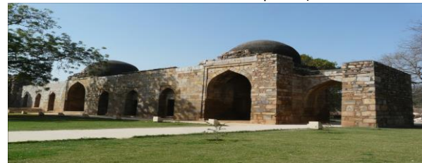
(Figure13: northwest rooms of Alai madrasa)
