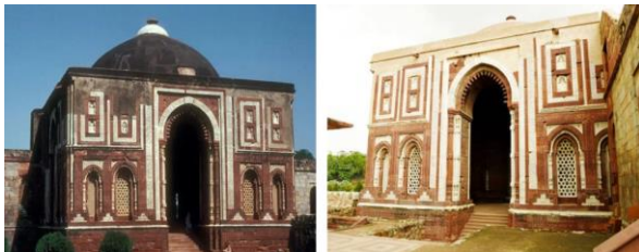
(Figure10B: Western entrance and eastern entrance)
